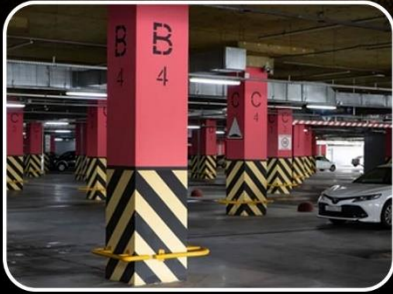
3 FLOORS COVERED CAR PARKING
